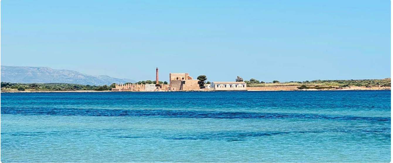
The Tonnara of Vendicari with the chimney and the tower by the sea
