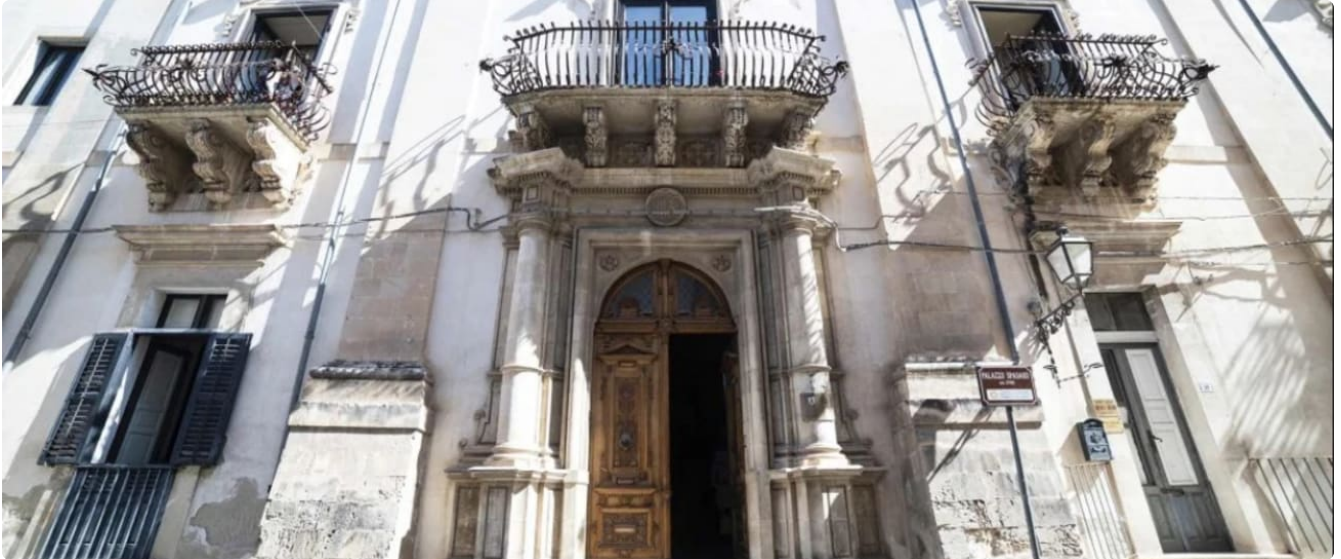
The wrought iron balconies of Palazzo Spadaro on Via Mormina Penna in Scicli
