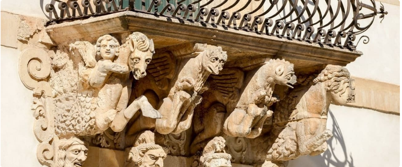
The balcony of the Grifi at Palazzo Fava, on Via San Bartolomeo in Scicli
