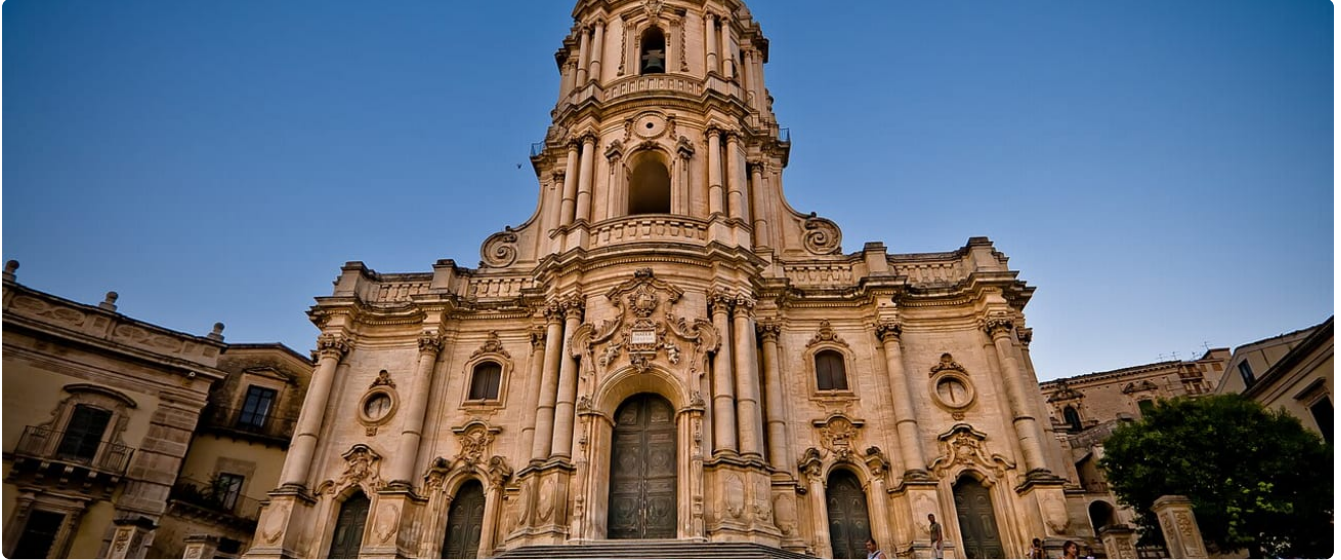
The tower façade and the staircase of the Cathedral of San Giorgio in Modica
