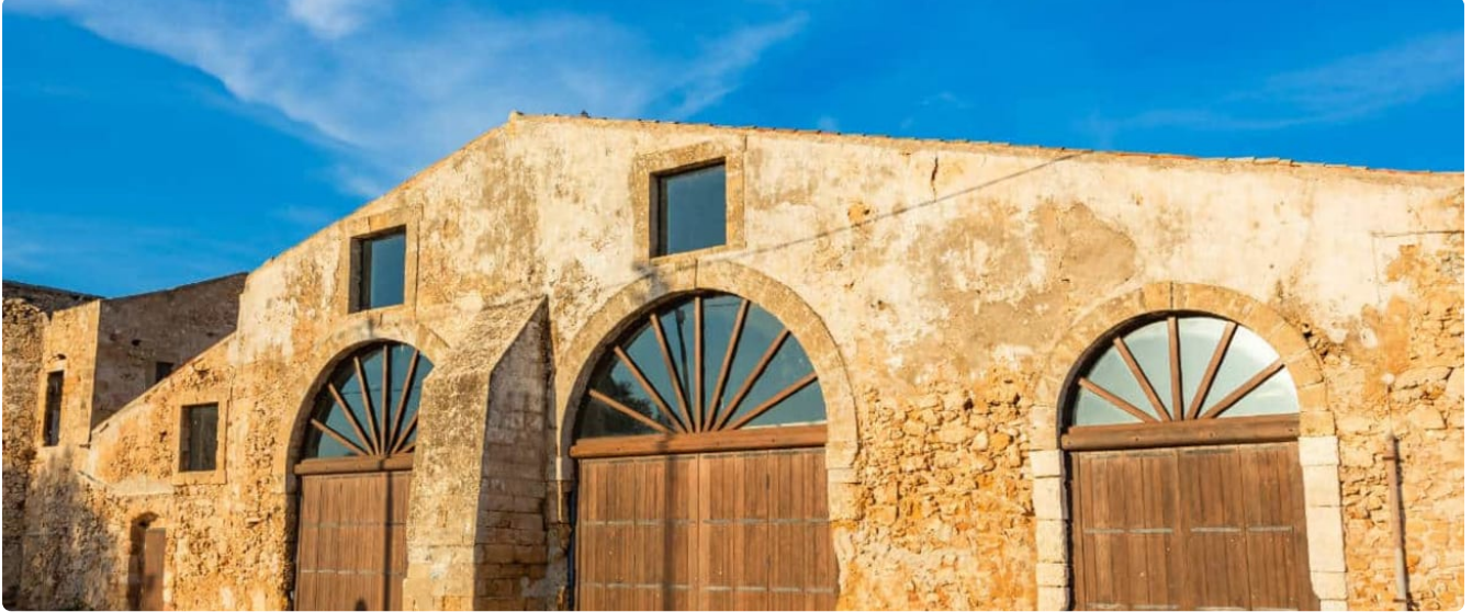
The loggia of the Scieri with the tuff arches and the sea, in the Tonnara of Marzamemi
